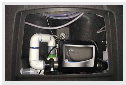
FIGURE 1.9: HEATER UNION; LOOSEN UP TO BLEED AIR
