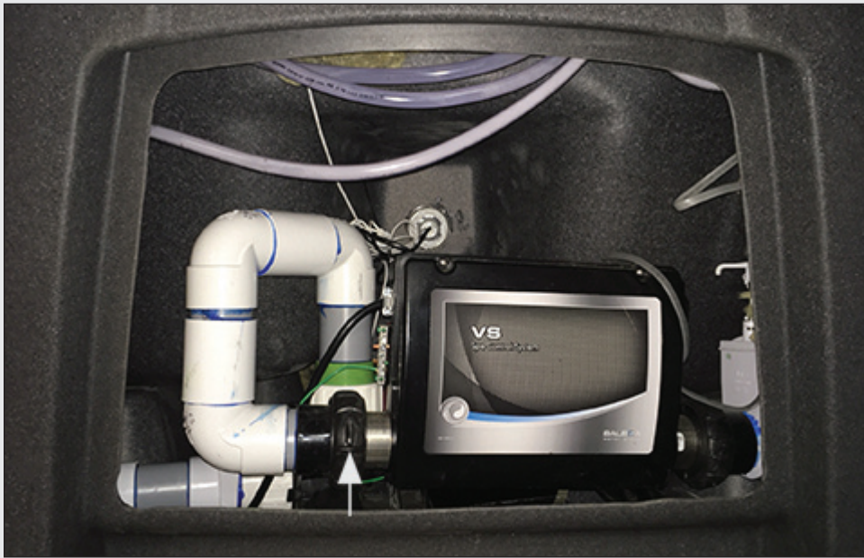
FIGURE 1.9 : HEATER UNION; LOOSEN UP TO BLEED AIR
