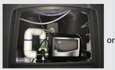
FIGURE 1.9a : HEATER UNION; LOOSEN UP TO BLEED AIR
