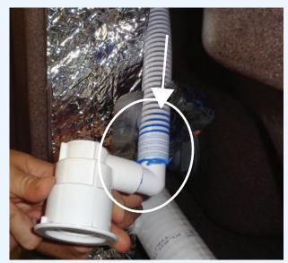
You must cut the hose just after the 90° adaptor. Please carefully notice the angle of the jet because when you will install the new one, it must be in the same direction;
