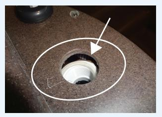
9 Replace the jet in the right place. Insert the flat gasket between the spa wall and the jet. Place the gasket with the groove facing the jet. Be sure to place the jet at the same angle as when you removed it;
